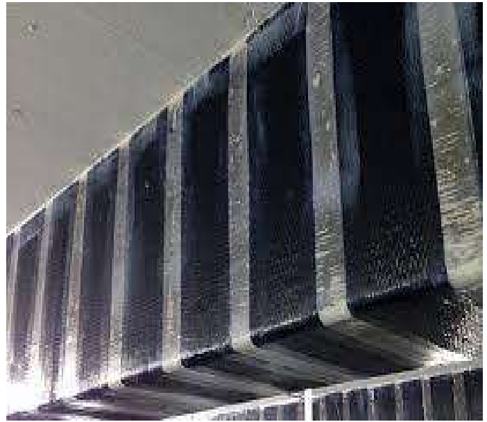
Fig. Carbin Fibre Reinforcement
