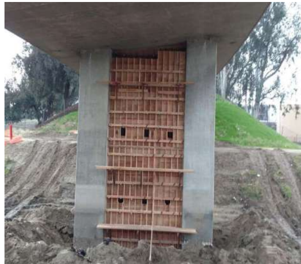
Fig.Retrofitting of a bridge
