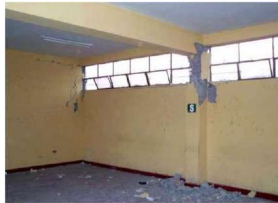
Figure 1.6: Damaged column [3]
