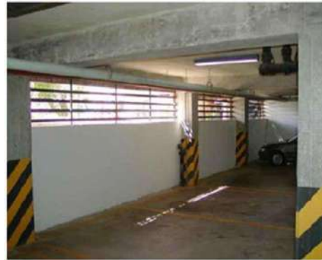
Figure 1.2: Partial infilled wall - short column formed [21]
